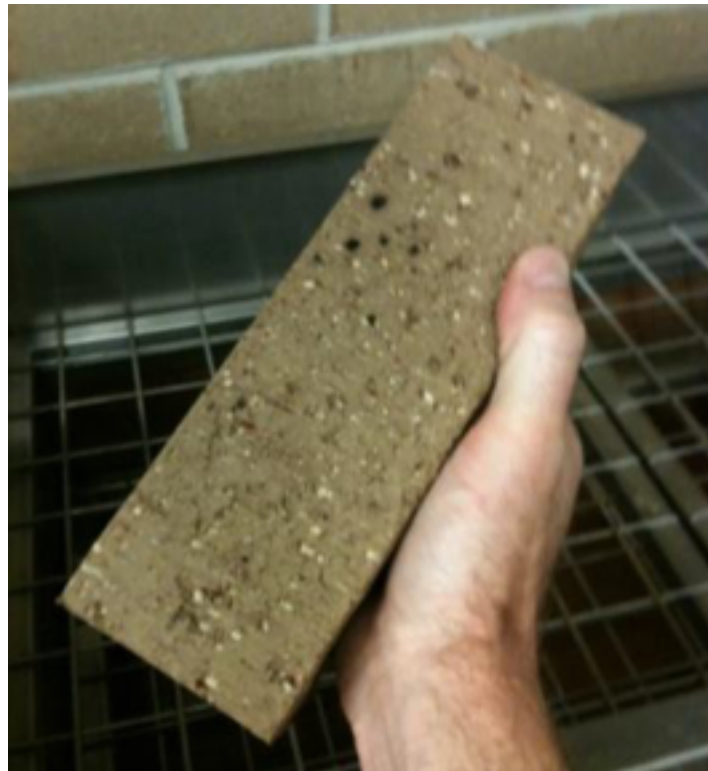
Assessment of lime pitting after steaming for moisture expansion assessment
