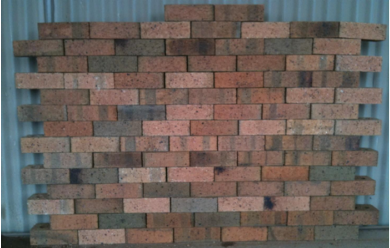
Of the 100 bricks in this wall only 4 showed visible cracking when viewed at 6.1 metres
