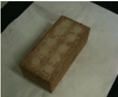
The cores of the brick are filled with sand
