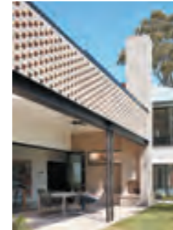
Tim Stewart Architects Mahara Street p.226
