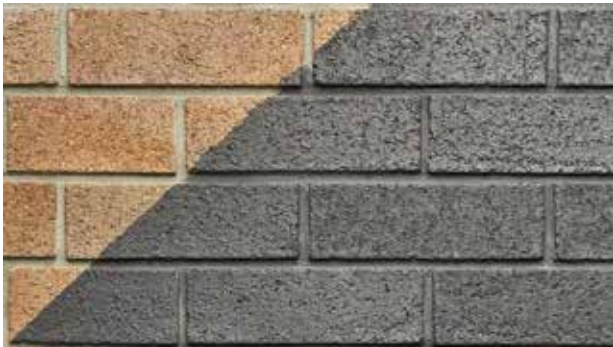
Paint Joint: Raked Feature: Paint Brick: Wire Cut Painter
