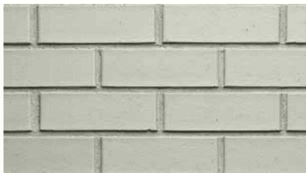
Paint Joint: Raked Feature: Paint Brick: Smooth Painter
